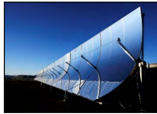
Figure 11 Outside Surface Absorber Technologies Without Cavity Receivers—Examples of Extreme Heat Loss, Low Temperatures & Inefficiencies (Line-Focus, BrightSource, AREVA)
