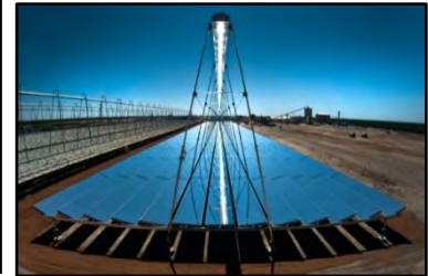
Figure 11 Outside Surface Absorber Technologies Without Cavity Receivers—Examples of Extreme Heat Loss, Low Temperatures & Inefficiencies (Line-Focus, BrightSource, AREVA)
